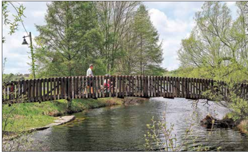
The Head Lake Park footbridge will be replaced with a Bailey bridge. Photo by Adam Frisk.
